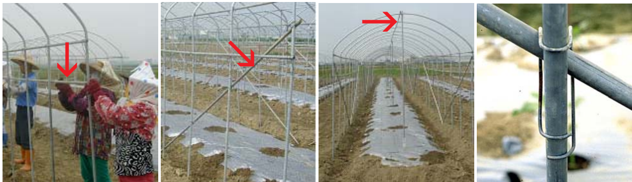
Fig. 6. Horizontal pipes, diagonal braces, and center top pipes are installed using steel clips.
