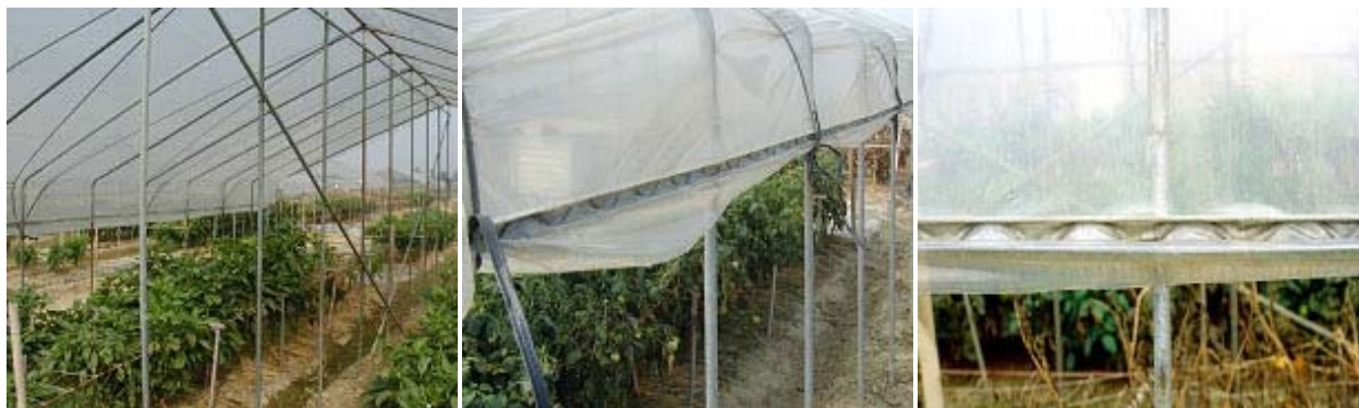
Fig. 10. Double-bed structures have center posts and their plastic covers are fixed against side braces with zig-zag wire clips.
