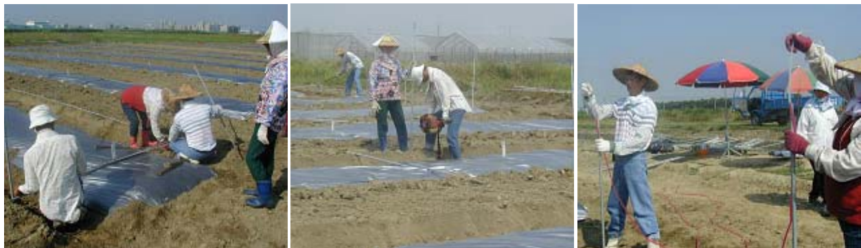
Fig. 5. Foundation posts are marked, holes for posts are drilled, and posts are leveled.
