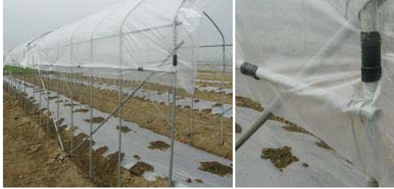
Fig. 7. The plastic cover is installed and then secured with plastic clips.
