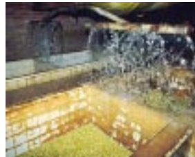
Fig. 4. Automatic sprinkler system with tile-lined germination tank
